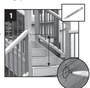
**NOTE:** If deck boards are not installed yet place an appropriate deck width spacer board to ensure post sleeve is at correct height.
