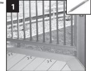
2. Drill a .9" (23mm) diameter hole 3/4" (1.9 cm) deep into deck board. Make sure hole does not go all the way through deckboard or light will fall through. Drill a 3/8" (8.25mm) diameter hole in base of the first hole through deck board making sure drill bit is perpendicular to board.
