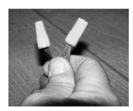
Step 8 Combine pigtail wires and additional wire if needed
