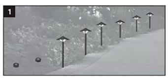
1. Locate placement of lights and lead wiring. If you choose to bury wire, under concrete or other permanent structures, plan accordingly.
