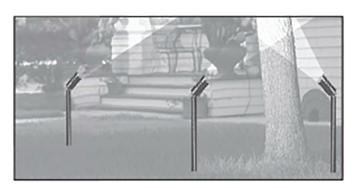
2. Place all lights in desired location. If necessary use 3/4" auger with in a drill to penetrate the surface enough to ensure the fixture is firmly implanted. **BEFORE YOU DIG - CALL 811**
