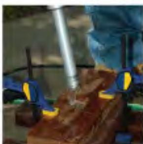
Turn on water at valve, hold at 45° angle start drill and set on paver
