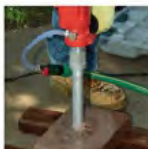
As drill bit gets started, straighten to 90°
