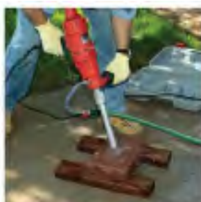
Turn on water at valve, hold at 45° angle start drill and set on paver
