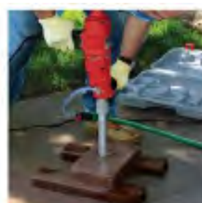
add pressure and drill through paver.
